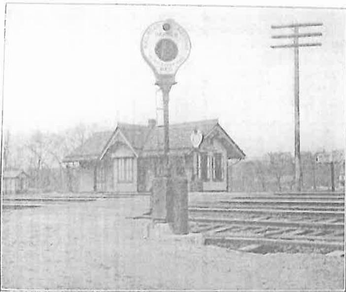
Audible and Two-Indication Visual Signal for Highway Crossing
